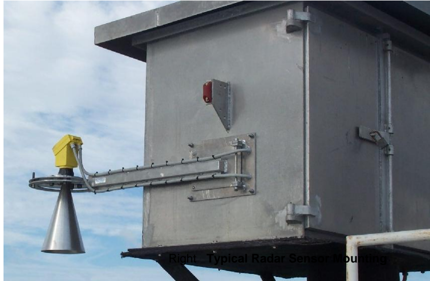
Typical Radar Sensor Mounting Environmental Protection Agency
