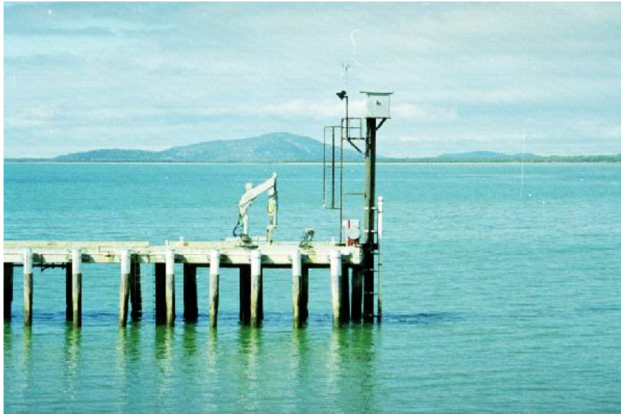
C Ferguson Storm Tide Station Environmental Protection Agency
