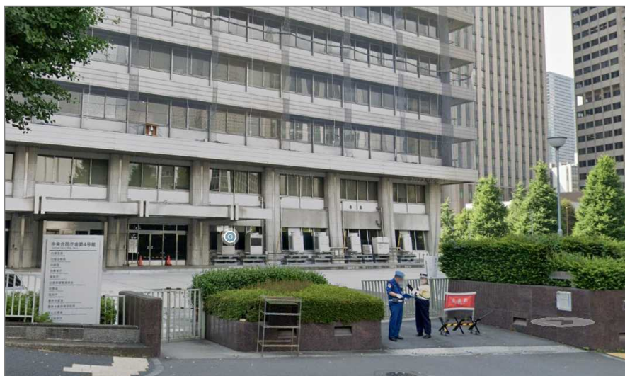
Entrance of the Central Government Building No.4 (South gate is “NOT” available for guests’ entry)
